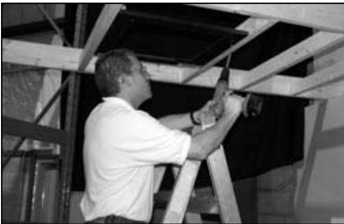
Figure 3: Attaching PIR to blocking.
